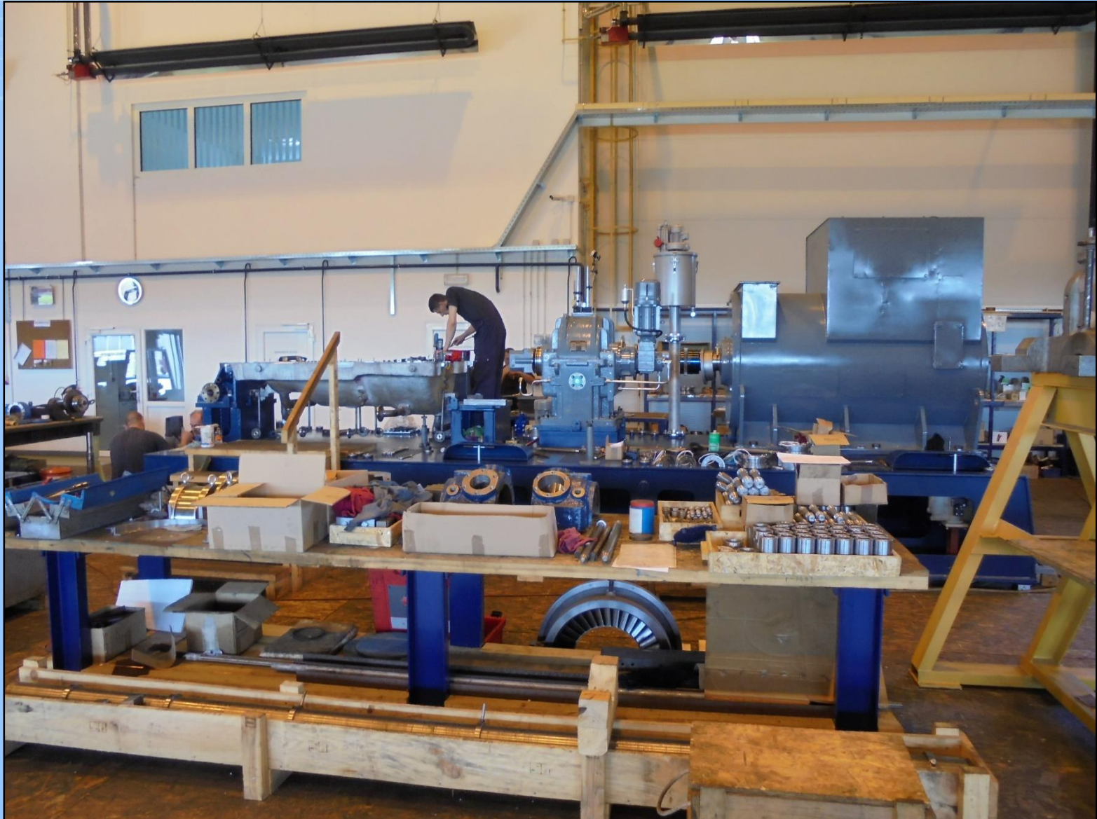
Montaža turbine 2,0 MWe BE-TO „SAVA” Stara Gradiška u TTK
